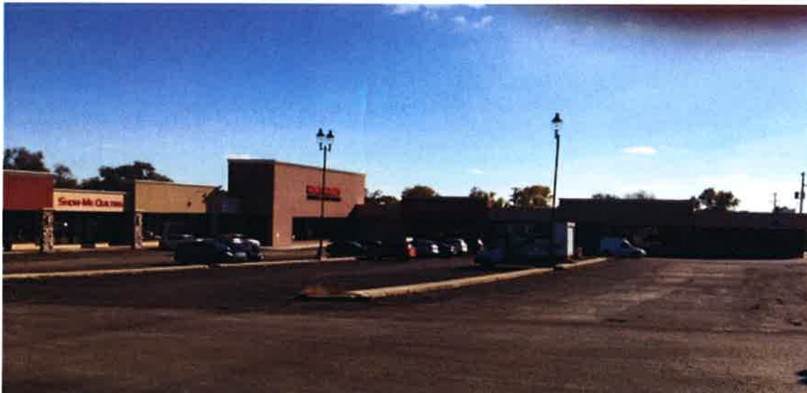
Figure 1 – View of South Building of Raytown Plaza Shopping Center
